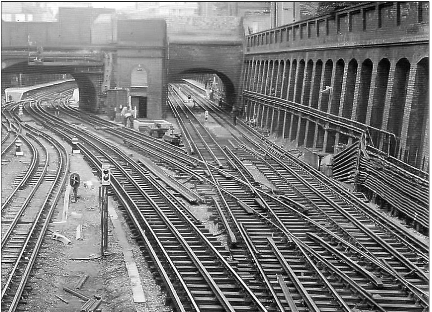
Above: Taken from the signal cabin east of South Kensington, this view looks west before the track rearrangements in 1957. On the left are two sidings, then the westbound and eastbound District Line tracks and then to the right, the outer and inner rail Circle Line tracks.
